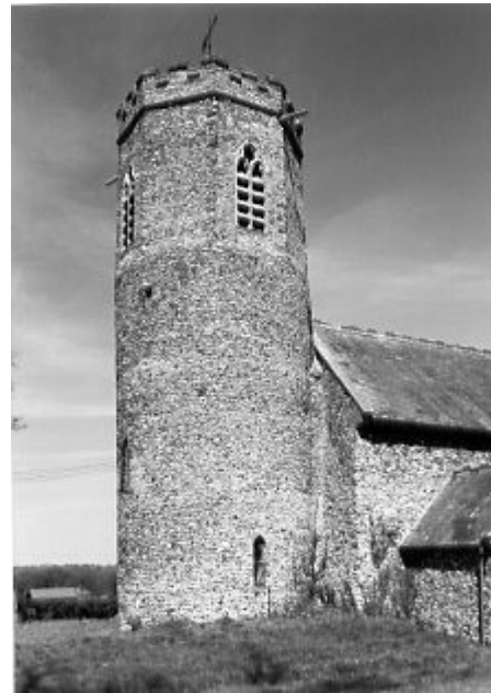
The tower from the south-west. Note the flint quoins at the south-west corner of the nave.
