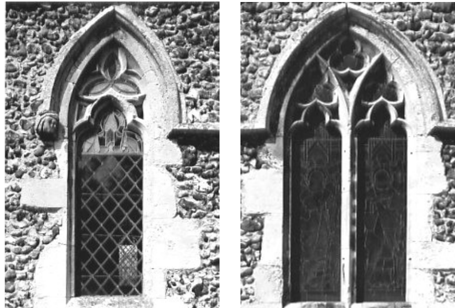
One of the lancets and the two-light Y-form window in the chancel south wall.
