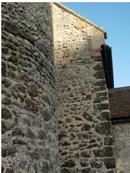
South west nave quoins worked from large blocks of iron-bound conglomerate.
