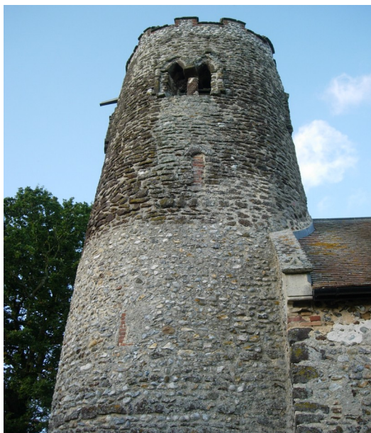
Bessingham round tower showing bands of iron-bound conglomerate near the base and used en-mass for the upper part of the tower.
