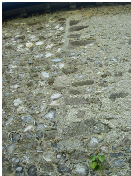
'Fossil' iron-bound conglomerate quoin line in the north wall of nave.
