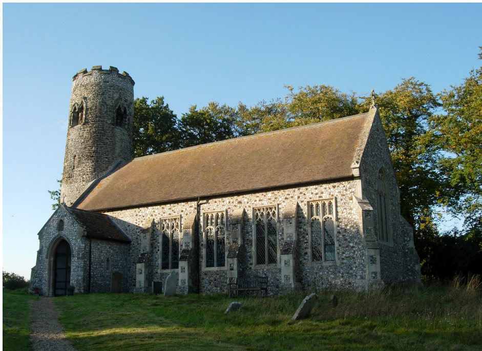
South wall of Bessingham church nave showing reuse of iron-bound conglomerate cobbles in a scattered pattern
