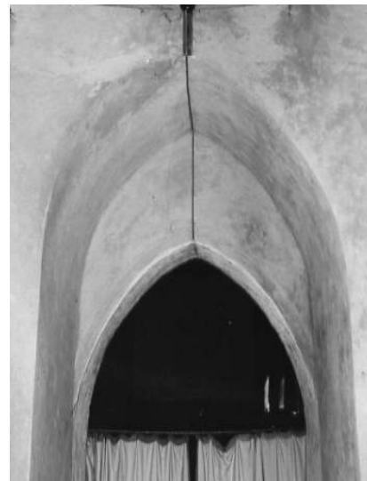
3. Ilketshall Sy Andrew. The tower arch in the tower, showing the separate arches in the nave and tower walls
