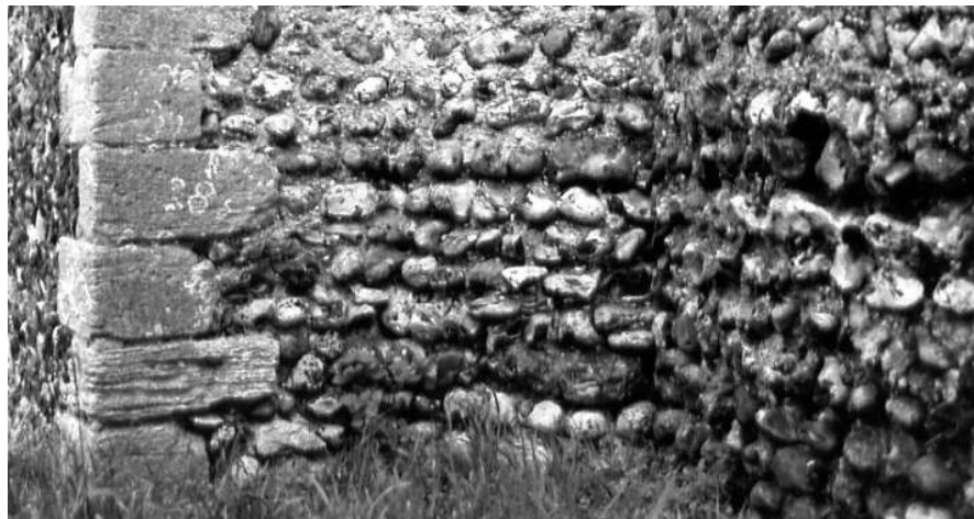
1. Quidenham. Coursed flints of the nave west wall, the re-entrant fillet and the curved tower wall, all laid in alignment
