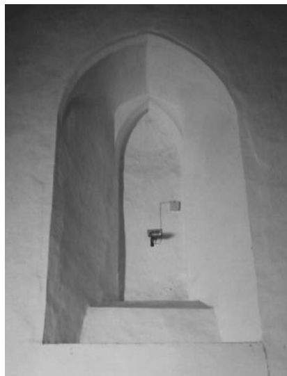
2. Welborne. Blocked former pointed window above the tower arch in the west wall of the nave
