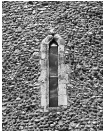
The south lancet window in the tower showing undisturbed flintwork around its stonework
