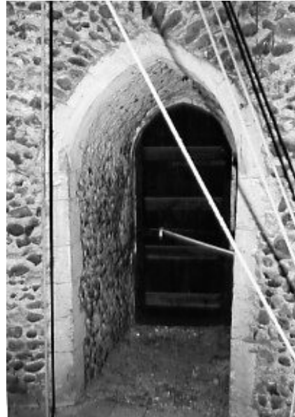
Upper door with pointed arch and stone dressings seen from inside the tower
