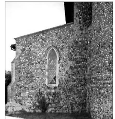
West walls of north aisle and nave showing uniformity of their flintwork
