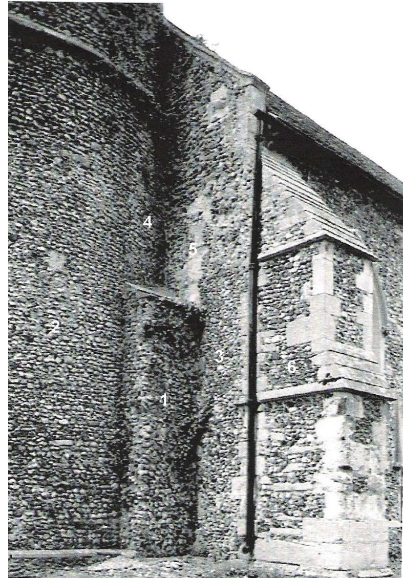
1997 photo of the SW corner, showing different building stages. See text.
