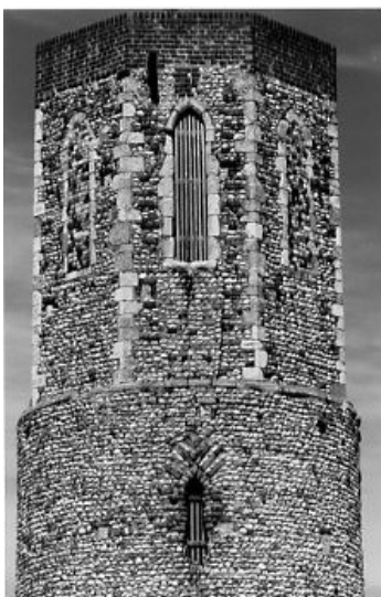
Upper part of tower before re-pointing
