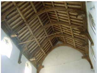
Hammerbeam roof
